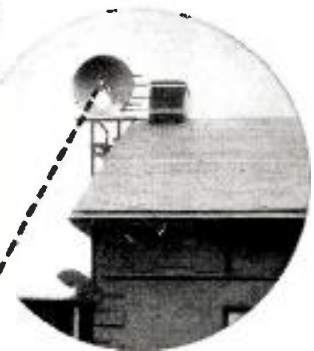
3. Simultaneously, the picture is transmitted by Federal microwave from an antenna on the station roof.
