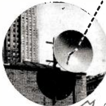
4. A similar antenna receives the picture at the LaSalle Street Union Station and feeds it to another monitor there.
