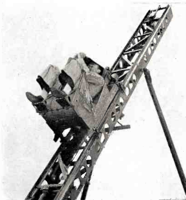
All in a day's work for Navy jet pilots. Powder charge in jet ejection seat model simulates the experience of rescue-ejection from a jet plane.
